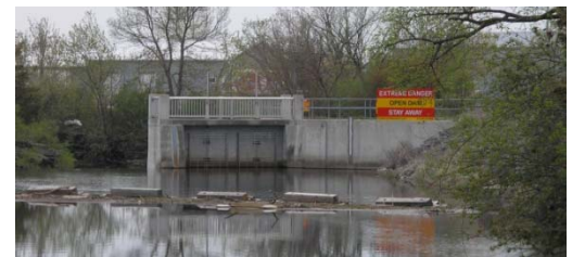
Figure: Low Head Weir underwater hydraulics, “drowning machine”. Sourced from Ministry of Natural Resource: Public Safety around Dams
