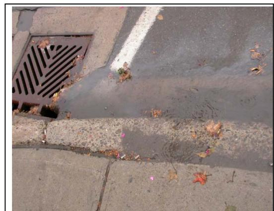
FIGURE 3: Local roadway runoff showing visible evidence of contamination
