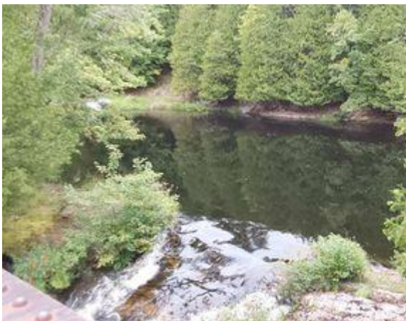
Photo 3: Looking Upstream from Structure
