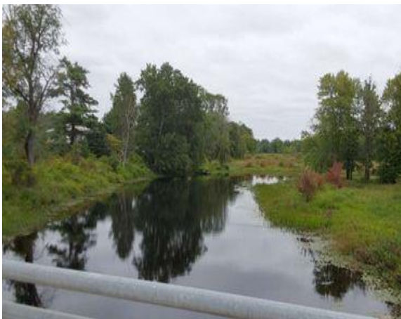
Photo 3: Looking Upstream from Structure
