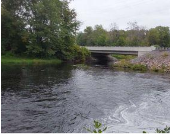
Photo 1: Upstream End of Structure
