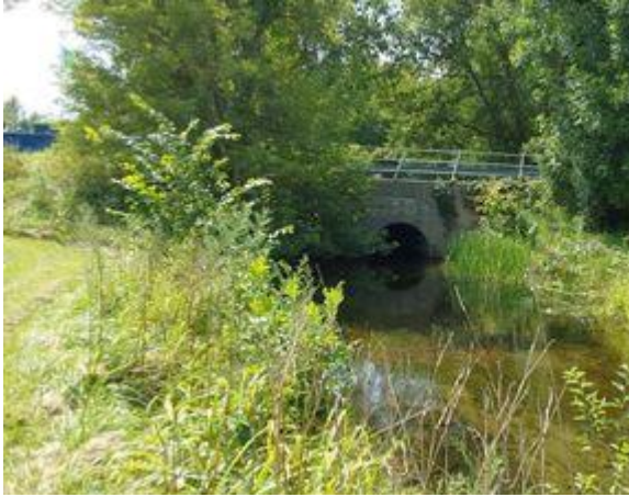
Photo 1: Upstream End of Structure
