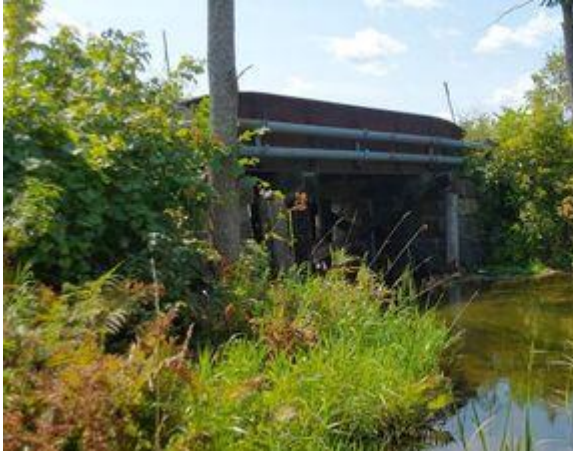
Photo 1: Upstream End of Structure
