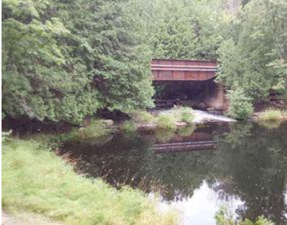
Photo 1: Upstream End of Structure
