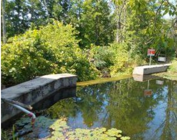
Photo 1: Upstream End of Structure
