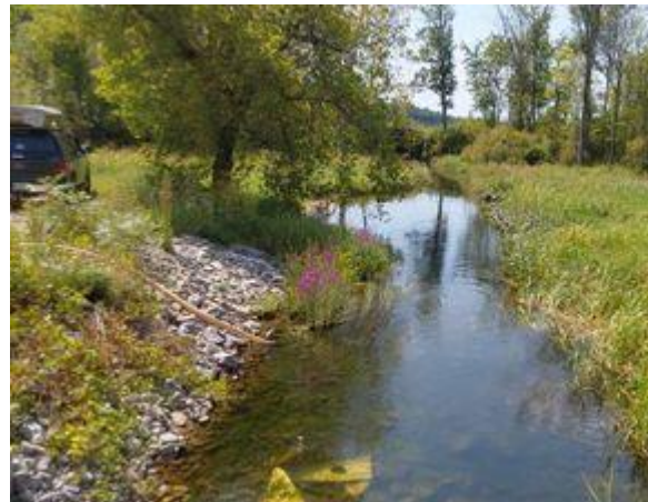
Photo 4: Looking Downstream from Structure
