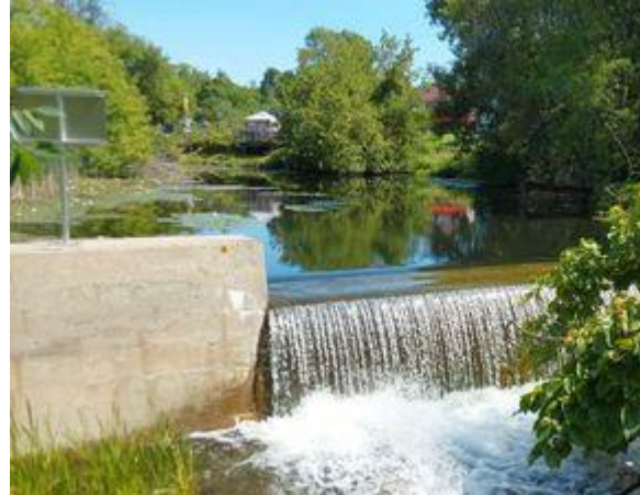
Photo 2: Downstream End of Structure
