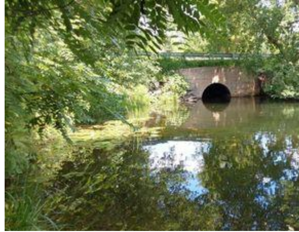
Photo 2: Downstream End of Structure
