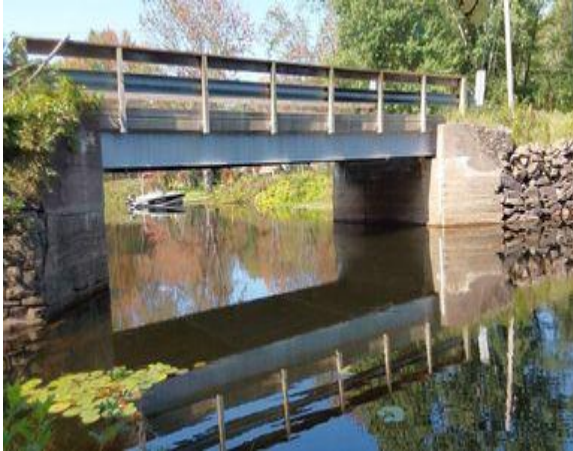
Photo 1: Upstream End of Structure
