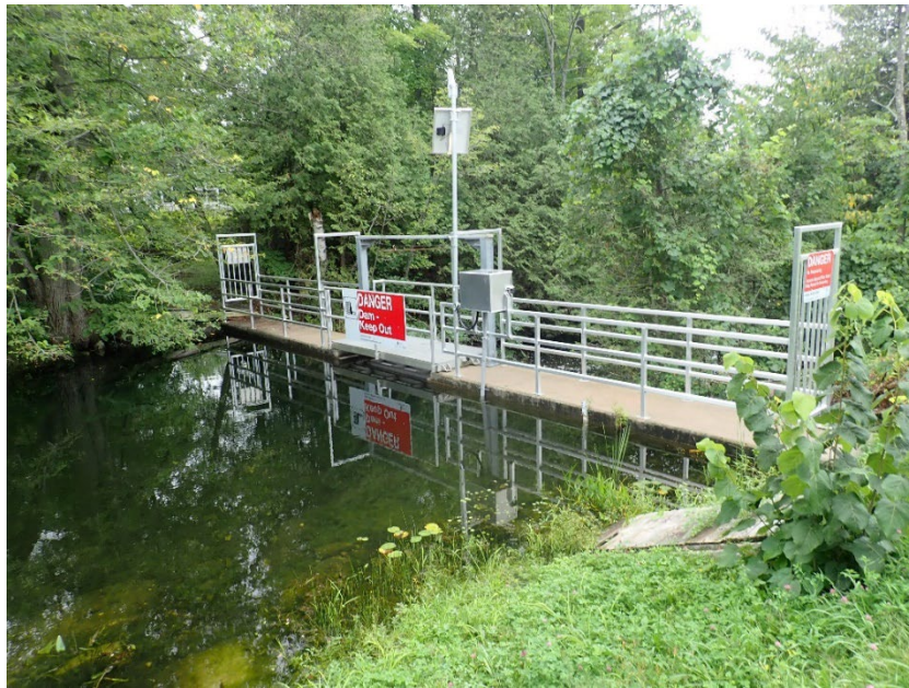
FIGURE 3-2: UPPER ARDEN DAM
