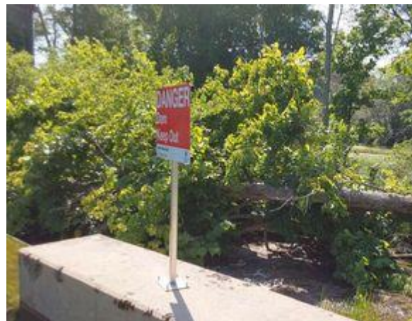
Photo 4: Looking Downstream from Structure
