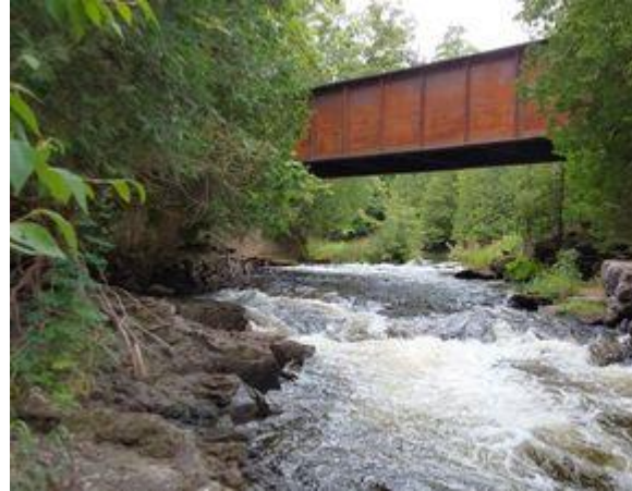
Photo 2: Downstream End of Structure
