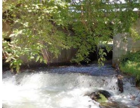
Photo 2: Downstream End of Structure
