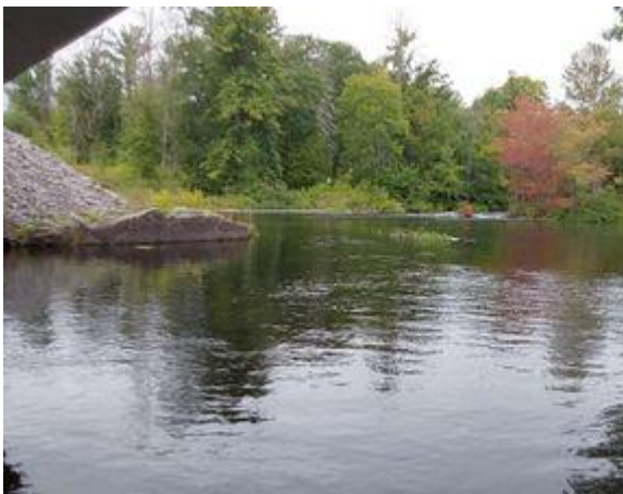
Photo 3: Looking Upstream from Structure
