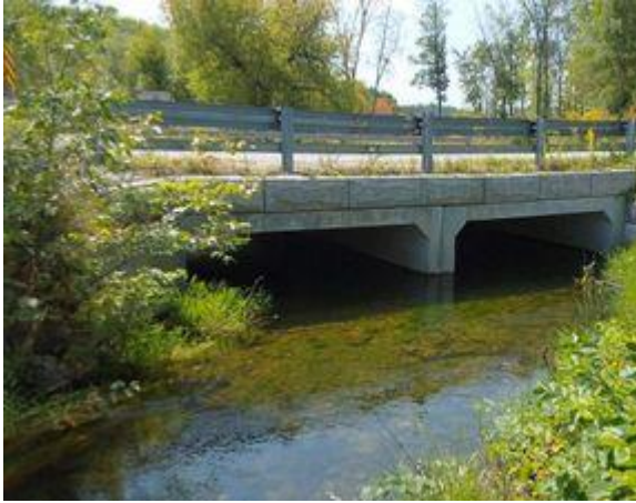
Photo 1: Upstream End of Structure
