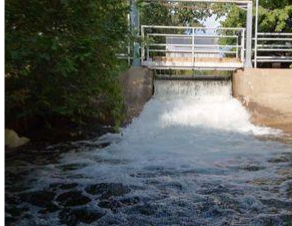
Photo 2: Downstream End of Structure
