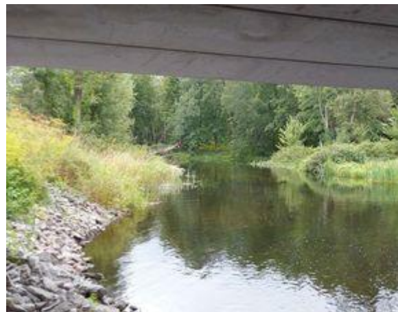
Photo 4: Looking Downstream from Structure
