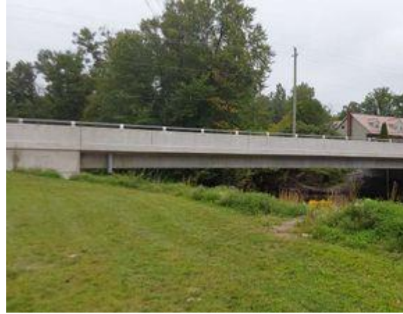
Photo 2: Downstream End of Structure
