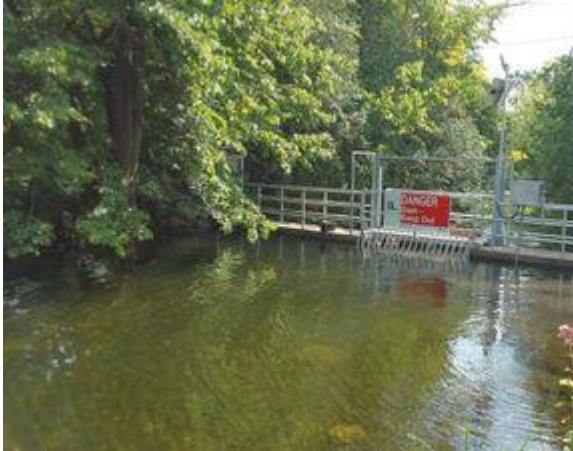
Photo 1: Upstream End of Structure
