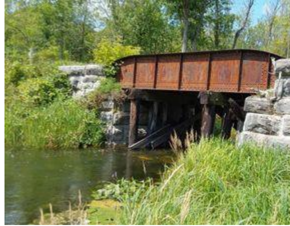
Photo 2: Downstream End of Structure
