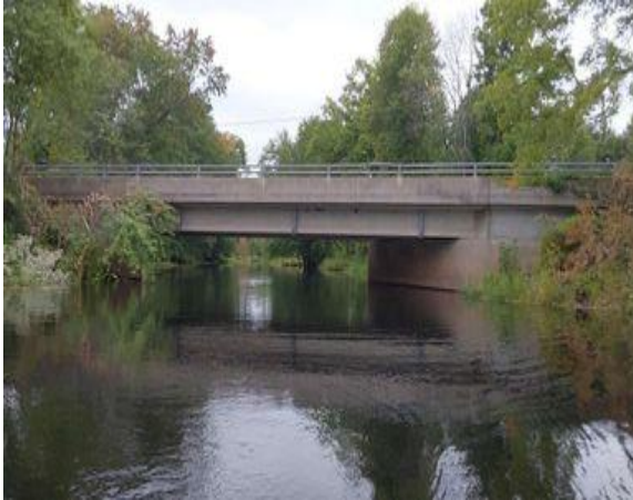
Photo 1: Upstream End of Structure
