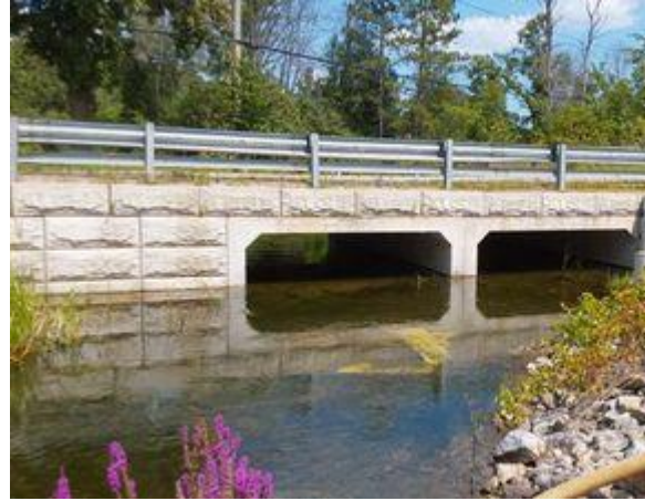
Photo 2: Downstream End of Structure
