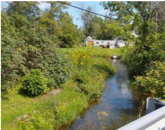
Photo 3: Looking Upstream from Structure
