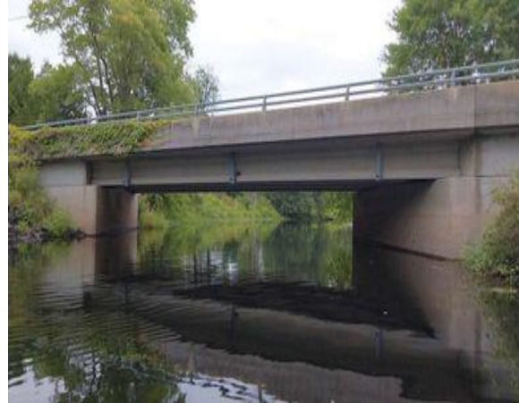
Photo 2: Downstream End of Structure
