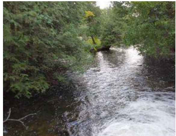
Photo 4: Looking Downstream from Structure
