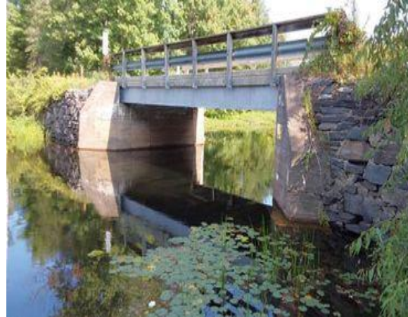
Photo 2: Downstream End of Structure
