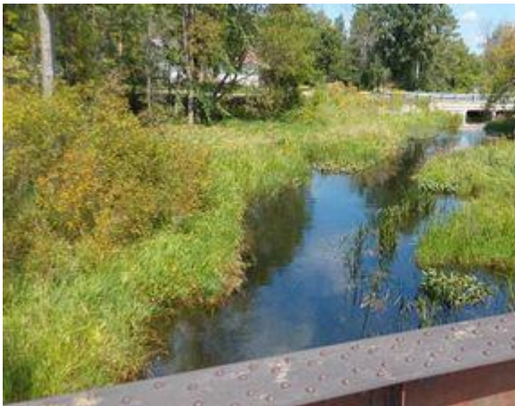
Photo 3: Looking Upstream from Structure
