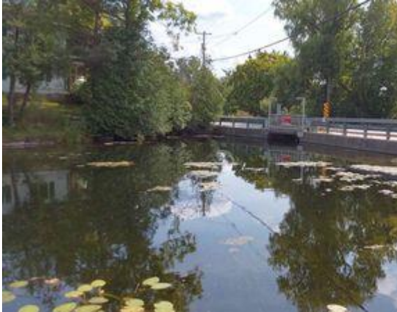
Photo 1: Upstream End of Structure
