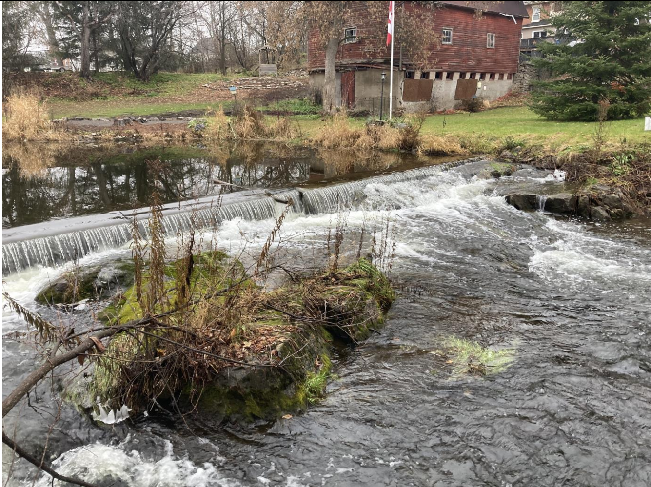
Figure 4-6: Photograph of the Weir/Drop Structure
