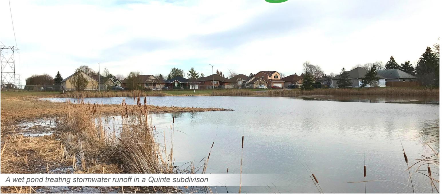
*A wet pond treating stormwater runoff in a Quinte subdivision*
