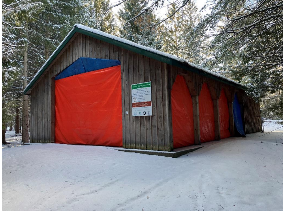
Figure 2.0 – North and West Wall of Pavilion.
