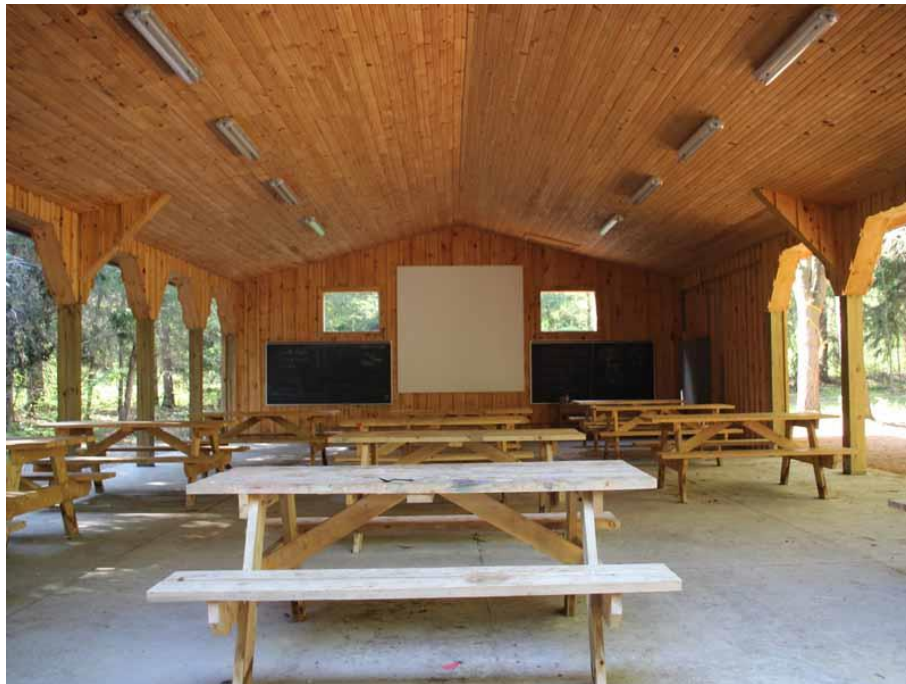
Figure 4.0 – Interior of Pavilion Looking South.
