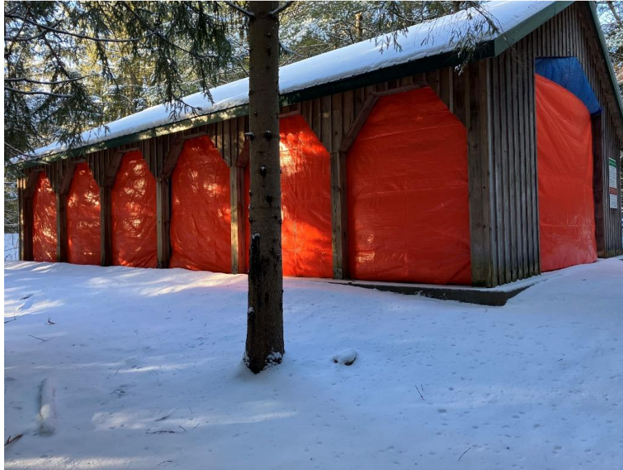
Figure 1.0 – East and North Wall of Pavilion.
