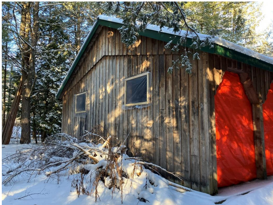
Figure 3.0 – South Wall of Pavilion.
