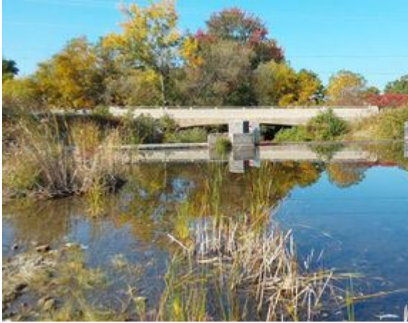
Photo 1: Upstream End of Structure
