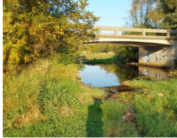
Photo 2: Downstream End of Structure
