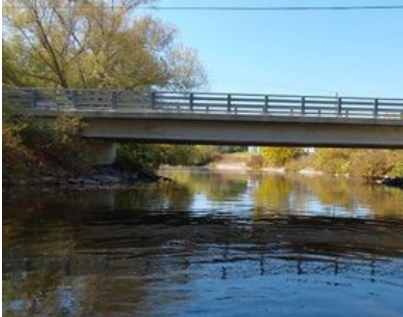
Photo 1: Upstream End of Structure
