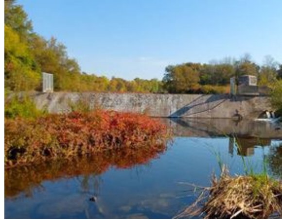
Photo 2: Downstream End of Structure
