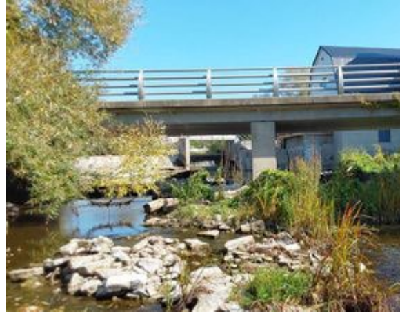
Photo 2: Downstream End of Structure
