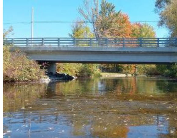
Photo 2: Downstream End of Structure
