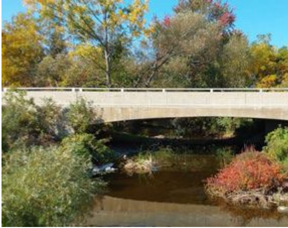
Photo 1: Upstream End of Structure
