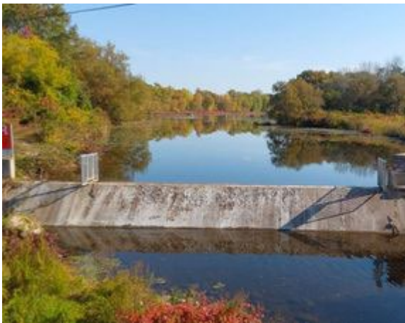
Photo 3: Looking Upstream from Structure
