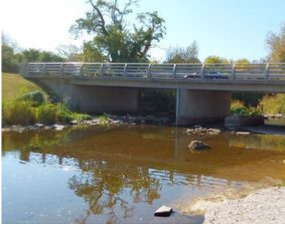
Photo 1: Upstream End of Structure
