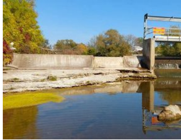
Photo 2: Downstream End of Structure
