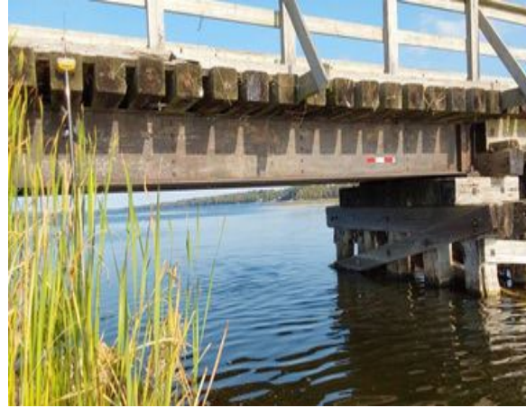
Photo 2: Downstream End of Structure
