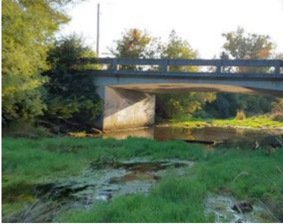
Photo 1: Upstream End of Structure
