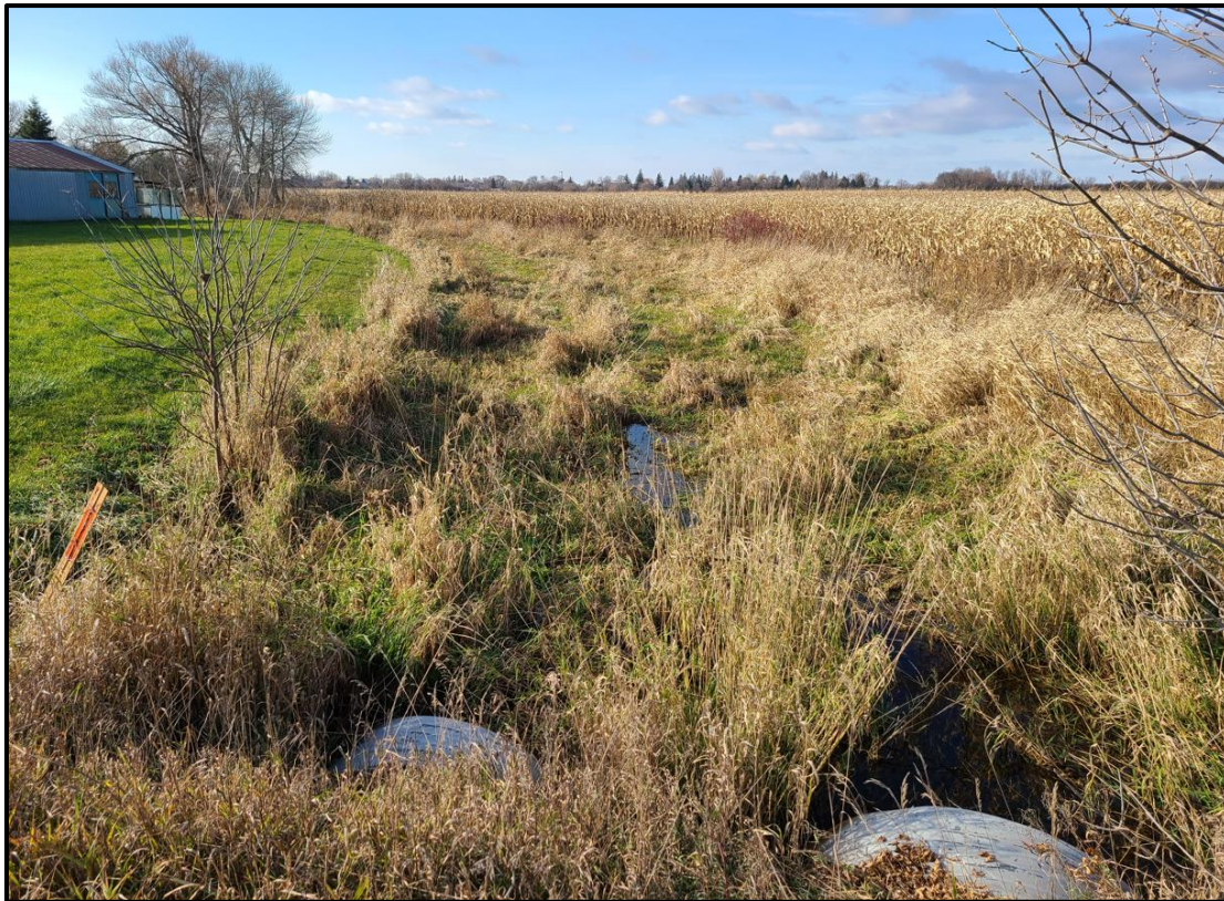
Figure 3-4: Image of Belleville Street Crossing Looking West
