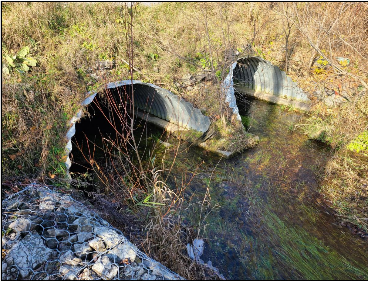
Figure 3-14: Image of Lake Breeze Court Culverts Looking West
