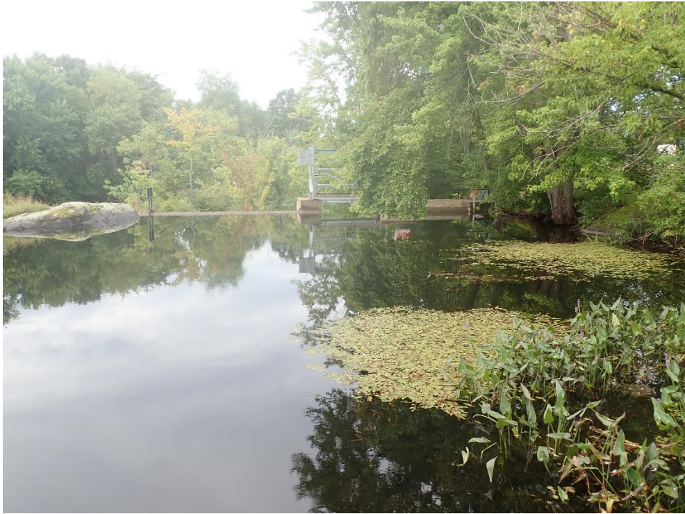
Figure 3: Looking at head pond and dam from upstream cattle bridge.
