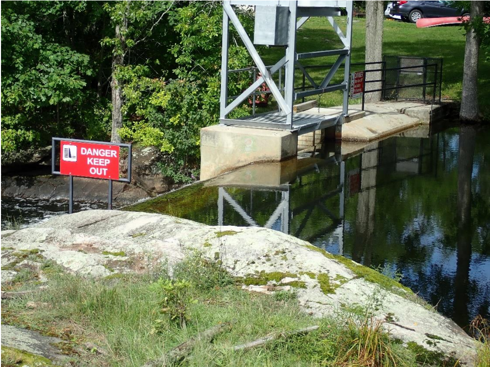
Figure 2: Looking at upstream side of dam from left bank.
