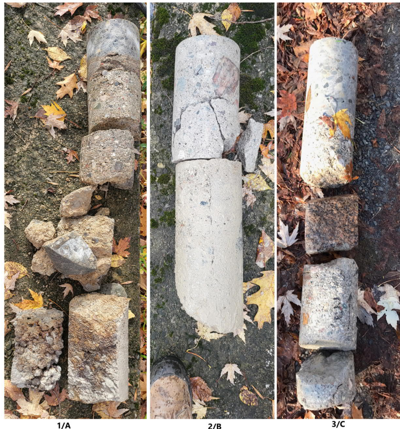
Figure 2-1: Three Concrete Cores Taken from Bellrock Dam
