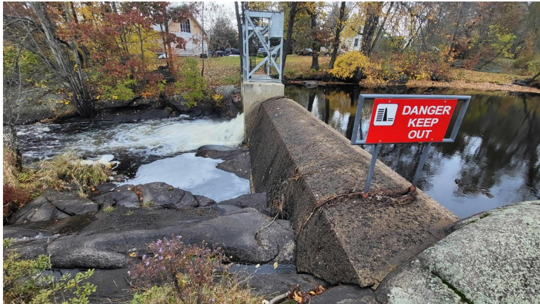
Figure 1-1: View of the Bellrock Dam
