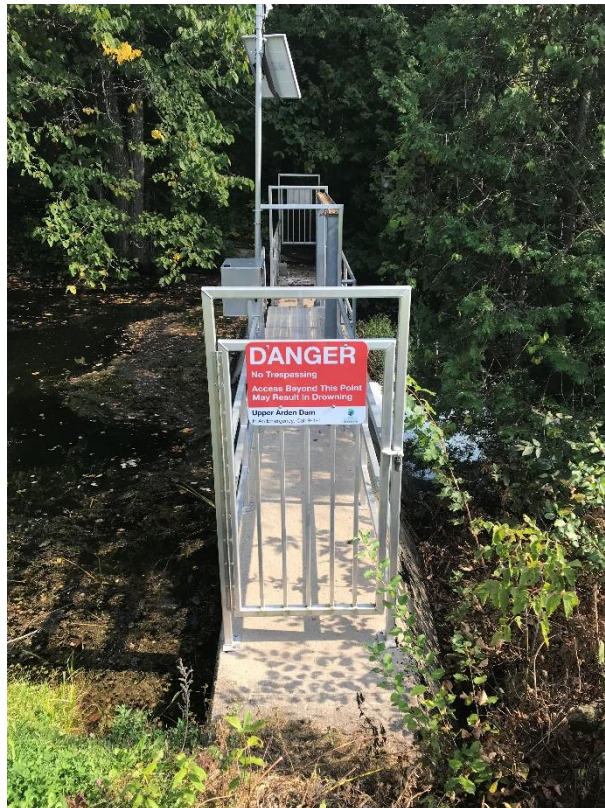
Figure 2.2: Upper Arden Dam, Dam Crest from Right Bank, 2024
