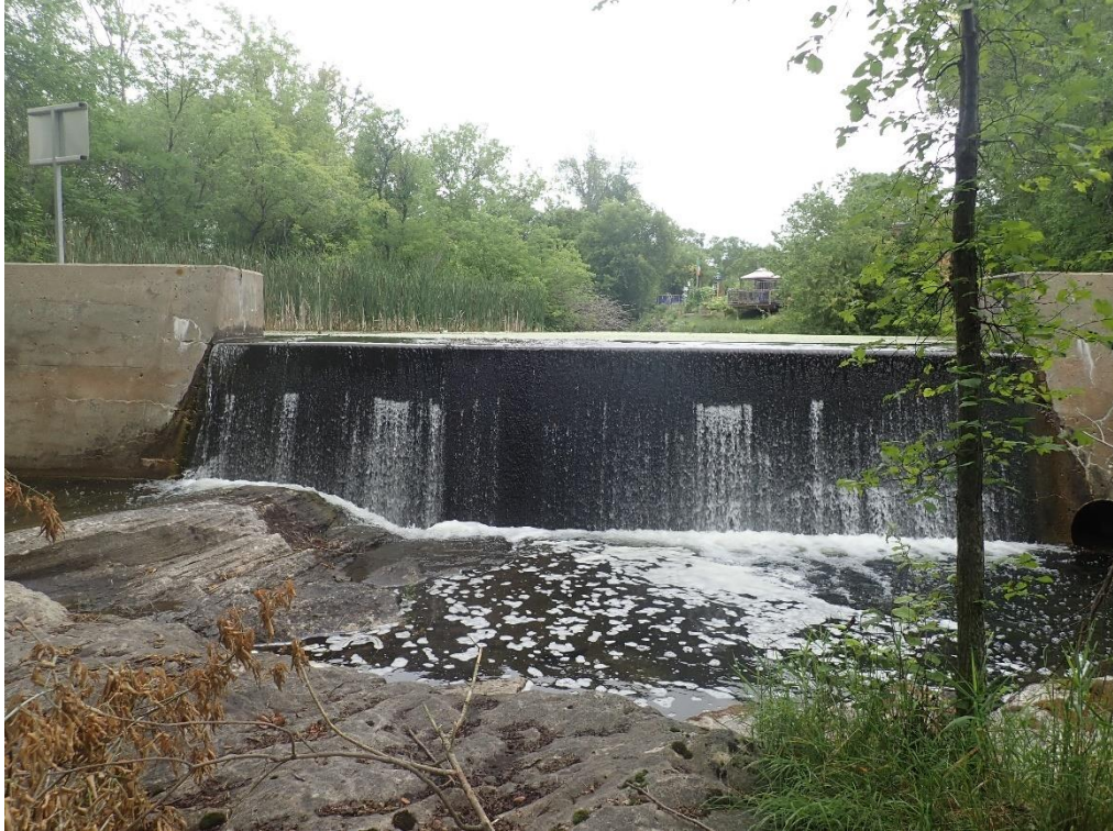
Figure 3.1: Lower Arden Dam, Spillway from Downstream of Dam, 2021
