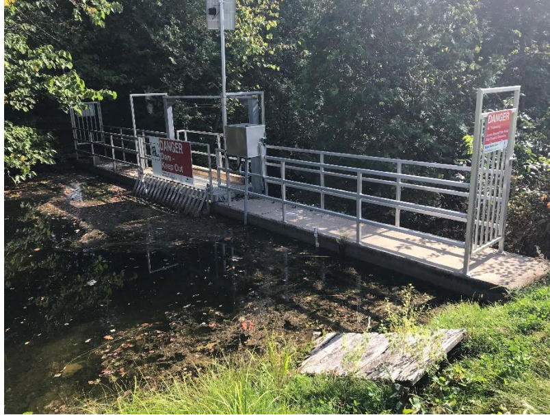
Figure 2.1: Upper Arden Dam, Upstream Side from Right Bank, 2024
