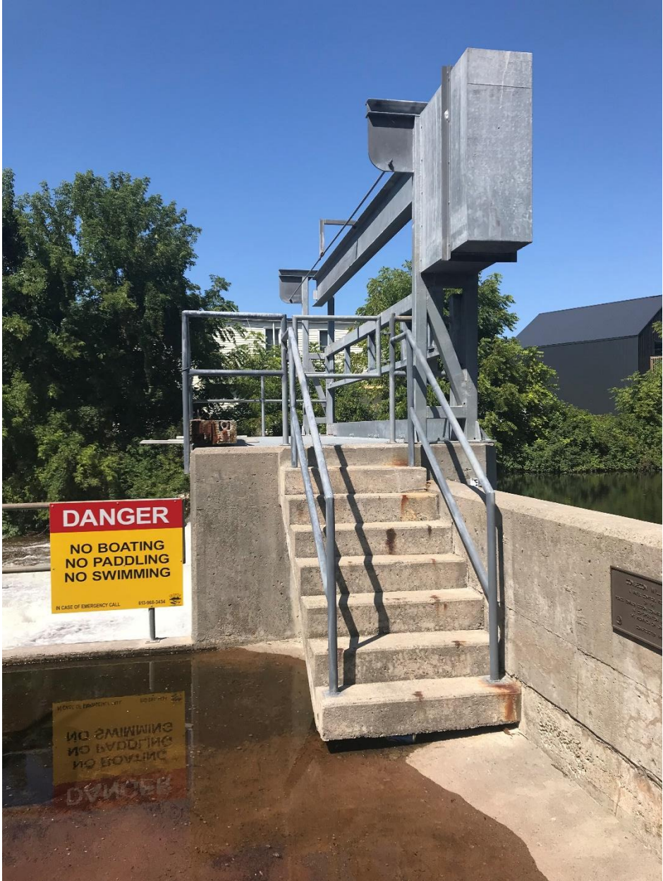
Figure 1: Stairs – Looking North
