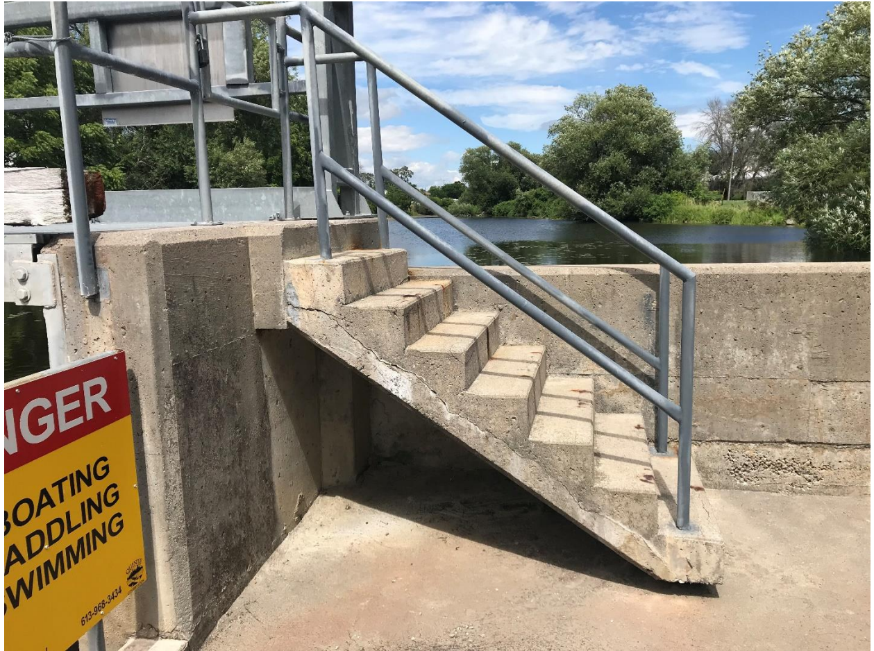
Figure 2: Stairs – Looking East
