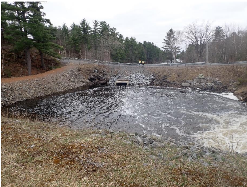
Figure 2: Standing on Embankment looking downstream at Roading/Culvert during high waters - 2018
