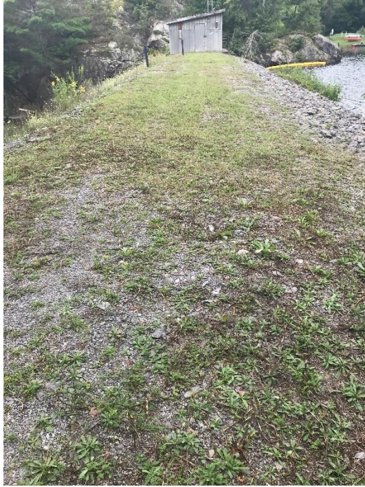
Figure 3: Looking at Outlet Gate House - 2023
