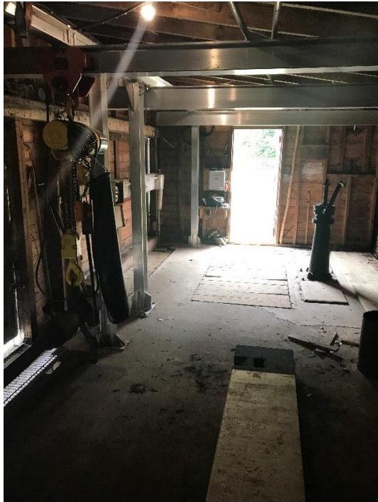
Figure 4: Inside Gate House
