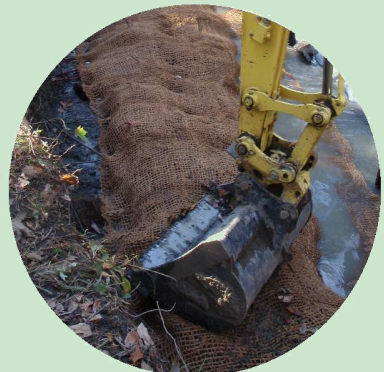
Coir fabric installation
