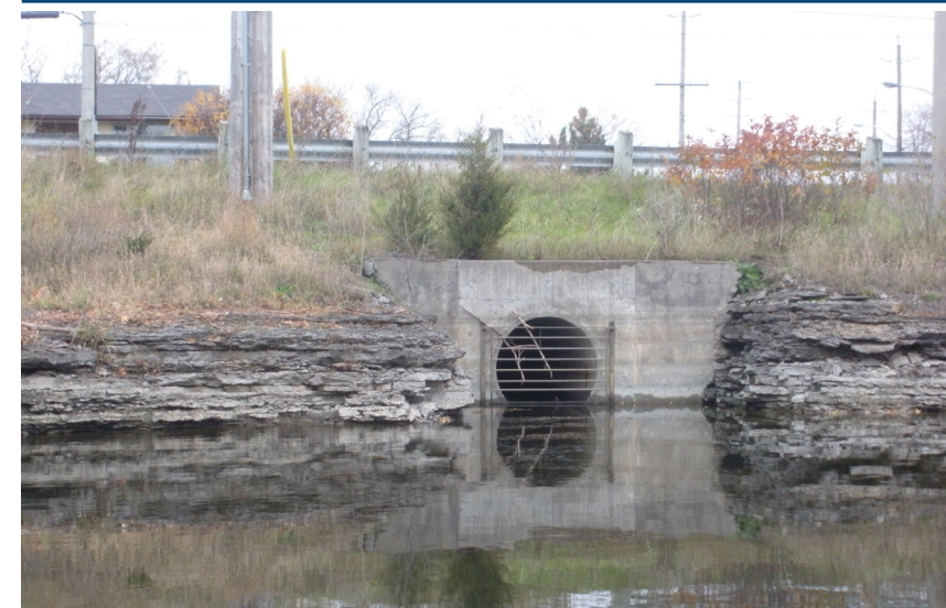
Stormwater Outfall
