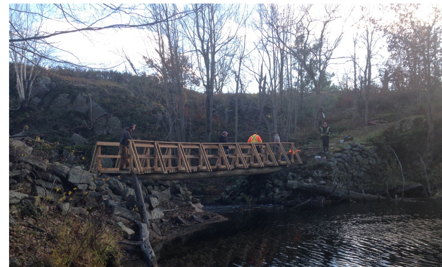
Workers replacing the bridge at Depot Lakes.
