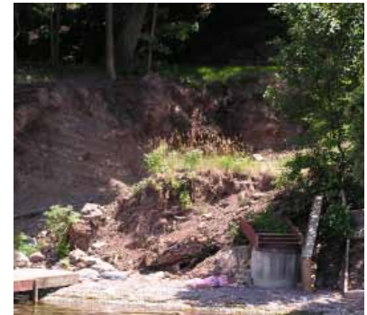
Above: Eroded Shoreline
