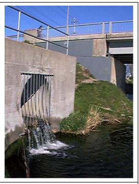
FIGURE 2: Some storm sewer outfalls may discharge continuously, even in dry weather. Above is 1650-mm pipe outfall to Trent River at Dixon Drive.
