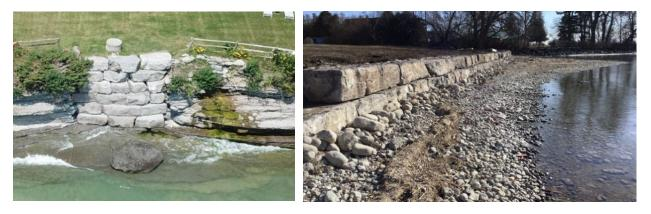
Figure 7.12 Stacked armour stone seawalls on Lake Ontario, "plugged" into an eroded section of bedrock cliff (left) and at the back of a cobble beach (right).
