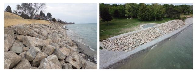
Figure 7.10 Examples of conventional, randomly placed armour stone (left) and field stone (right) revetments on Lake Ontario
