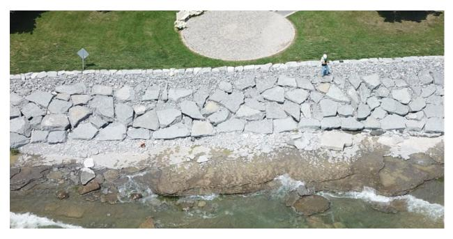
Figure 7.11 Single-layer blocky armour stone revetment with toe stones "keyed" into underlying bedrock shelf
