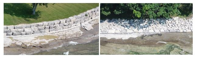
Figure 7.6 Example of conventional shoreline protection structures on bedrock shorelines; stacked armour stone seawall (left) and "keyed-in" armour stone revetment (right)
