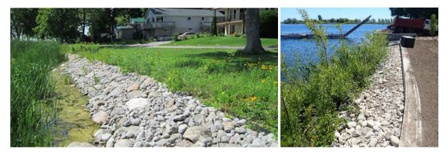
Figure 7.8 Hybrid grey-green shoreline protection structures featuring stone and/or concrete infrastructure fronted by vegetated natural buffers and natural riparian conditions
