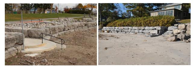
Figure 7.16 Examples of stacked armour stone beach curbs
