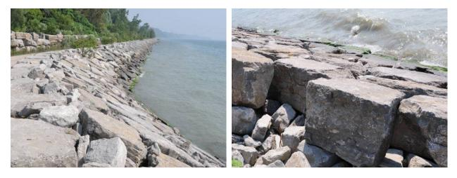
Figure 7.9 Examples of single-layer, blocky armour stone revetments on Lake Ontario
