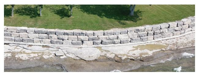
Figure 7.13 Stacked armour stone seawall founded on a thin concrete foundation over an irregular bedrock shelf
