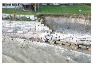
compared to their vertical counterparts. The adjacent image captured a vertical concrete block seawall failure on Lake Ontario during the high water period in 2017 and 2019.
